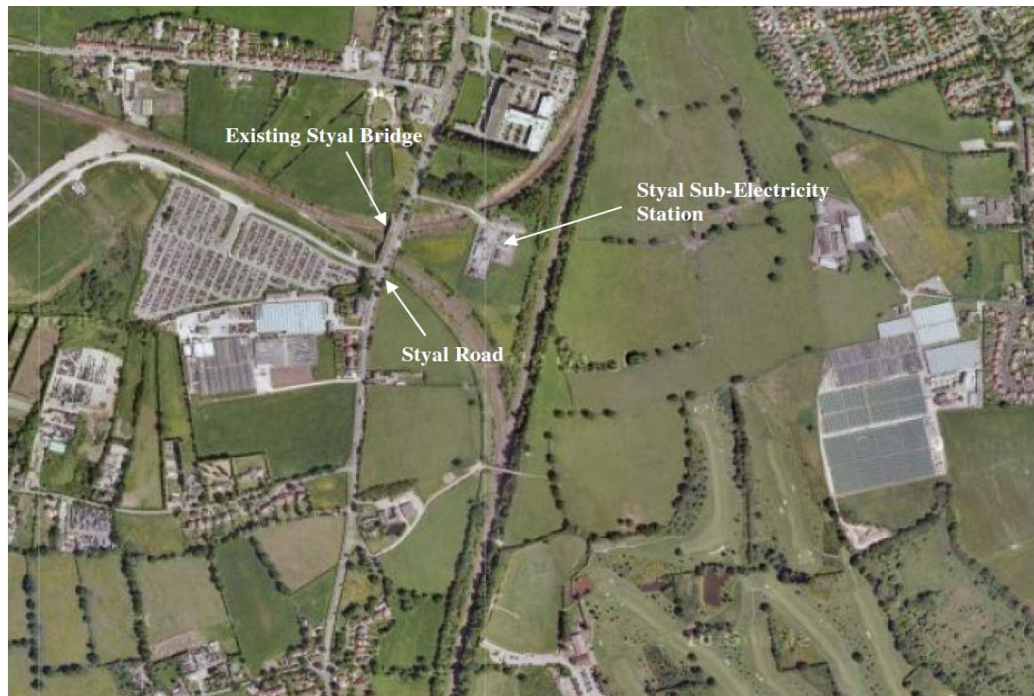
Top view of the bridge crossing
