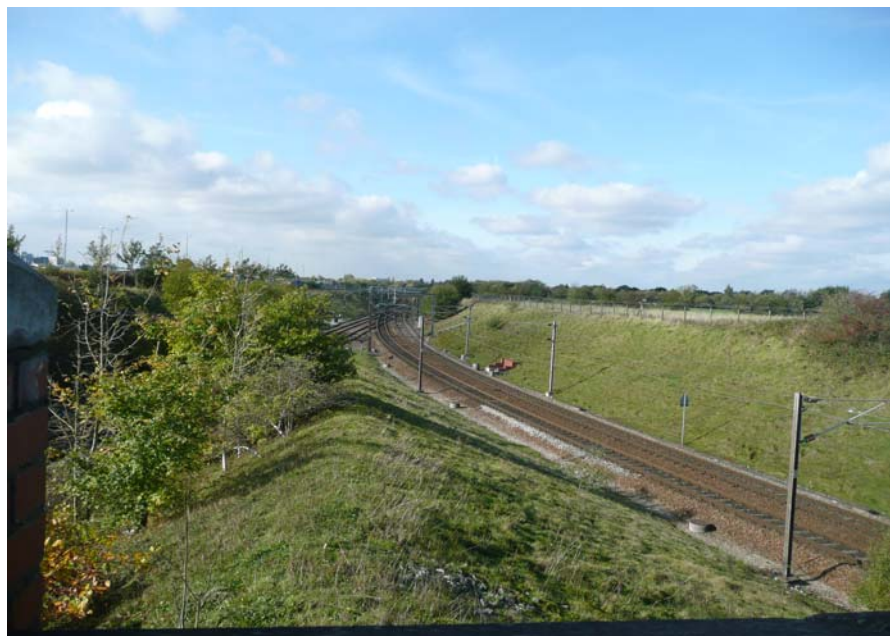
View showing the northern spur and the catenary
